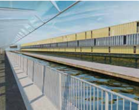
East Pier of Terminal
